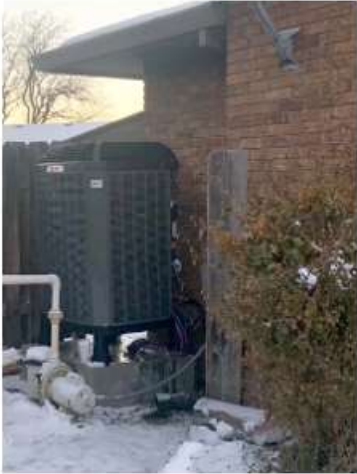
A Trane Heat Pump, July 2023.
