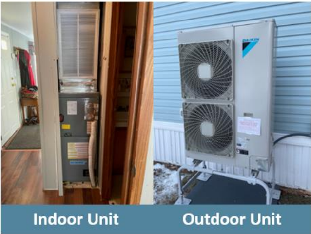
This is an example of what a heat pump system could look like on the inside and outside of your home.
